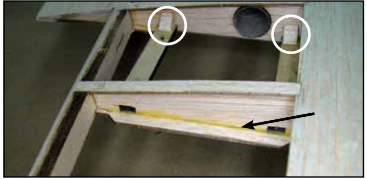
In the circles above are two gussets made from 1/4" triangle stock, use on both sides. The arrow in the lower part is indication the glue fillet between the cap strip and the rib.
