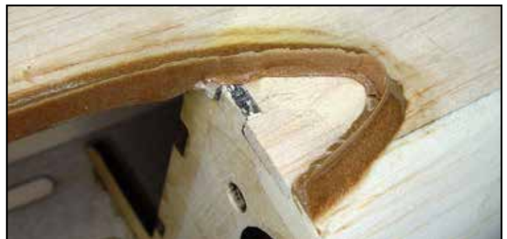
The feathered edge will be sanded smooth, note the fillet has been trimmed flush with the fuselage opening
